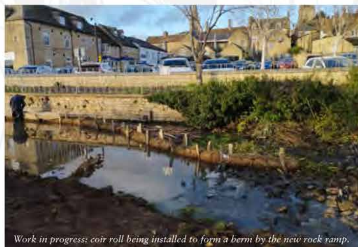
View of the millstream from the Lammas bridge after the works, showing planted coir roll installed on the concrete bank (with temporary protective structure) and recently regraded banks.
